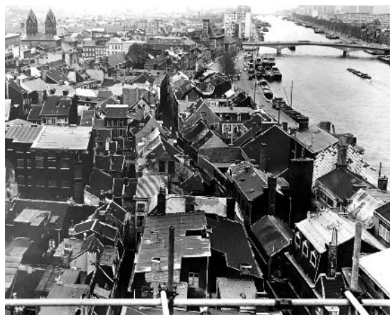
Figure 18 - View of the Saint-Georges district from the scaffolding of the new administrative centre, ca 1965 (CRMSF).
