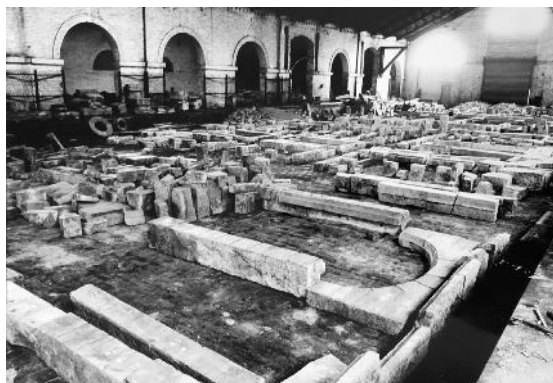
Figure 20 - View of warehouse where the dismantled facades are stored, waiting to be relocated (CRMSF)
