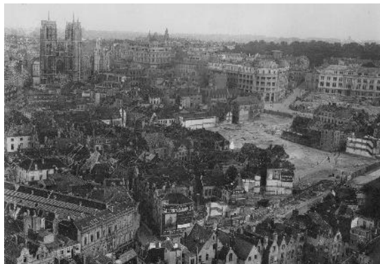
Figure 2 - The Putterie district seen from the tower of Brussels' city hall in 1912. Part of the area has already been demolished for the construction of the railway junction (© IRPA, a102953).
