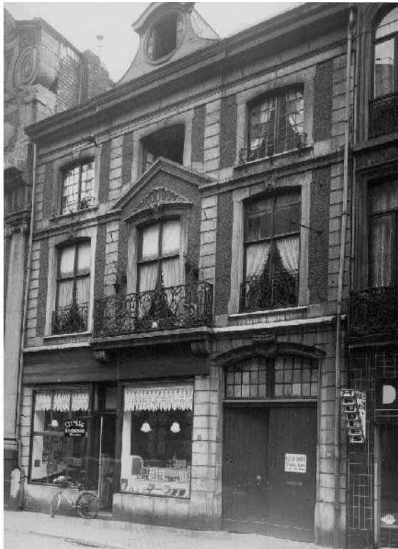
Figure 25 - House n°76, En Feronstrée, 1741-1760, demolished ca 1970 and relocated in the "archaeological block" (© IRPA, A017136).
