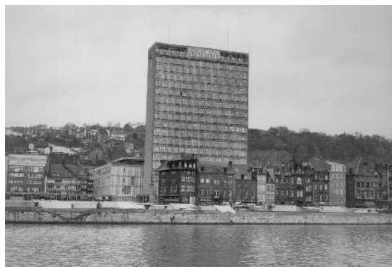
Figure 19 - View of the Quai de la Batte, the new administrative complex is in the centre-left of the image. the last building on the right will be relocated in the “archaeological block” (© IRPA, M043382)
