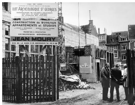
Figure 23 - The “archaeological block” under construction, ca 1975 (CRMSF)
